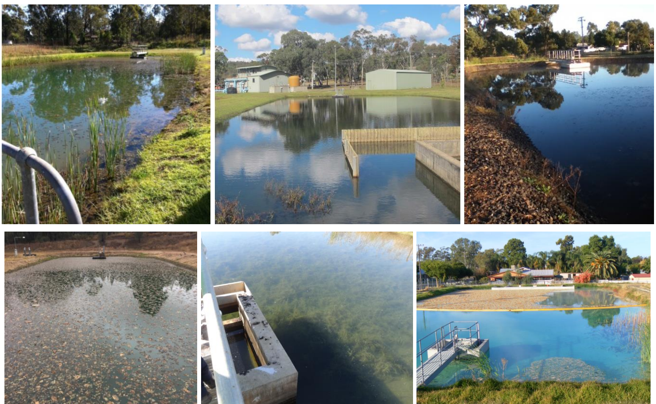
Figure 3-1: Examples of sedimentation lagoons (from left to right – Top – Binnaway, Coonabarabran and Mendooran WTP's in 2014, Bottom – Binnaway 2018, Mendooran 2017 and Coonamble 2018).
